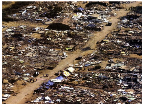
Figure 1: Bhachau Taluka Earthquake [1].
